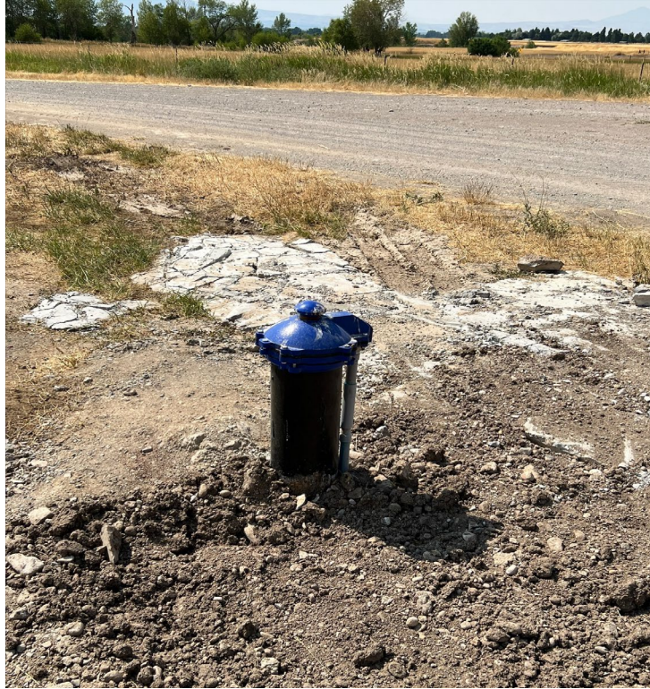
Photo 1 – New well installed in Spring/Summer 2024
