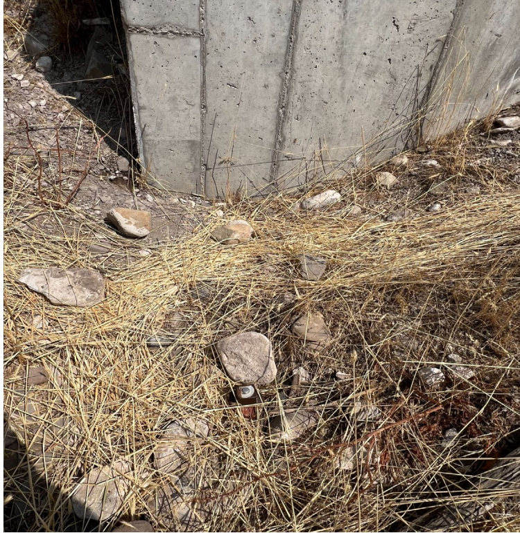
Photo 11 – Valve at cisterns (NW corner)
